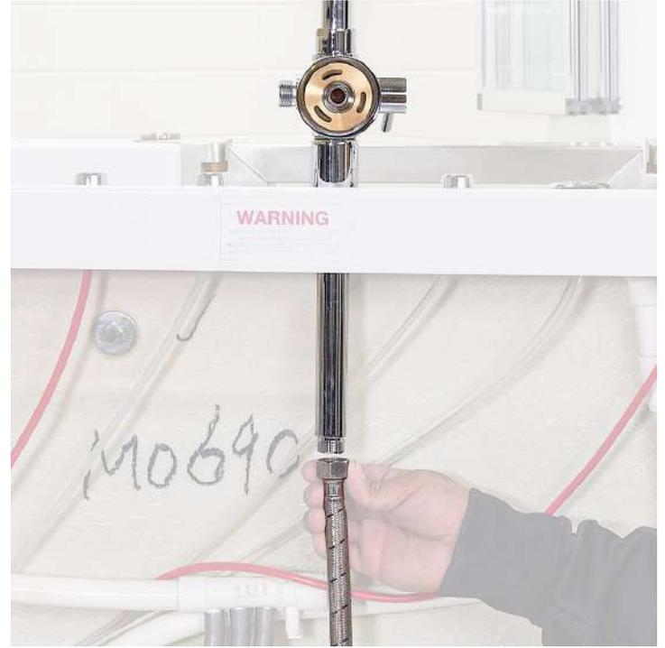
Tighten supply hose on the bottom of shower column
