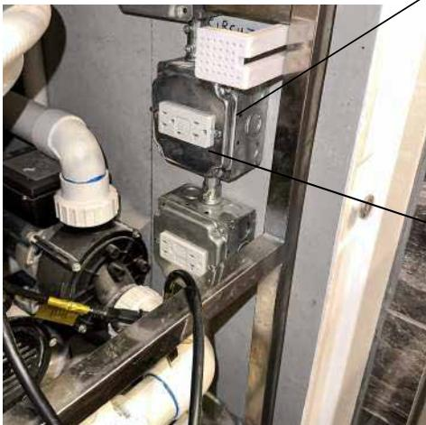
All electrical fixtures connect to a dedicated GFCI protected outlet or GFCI protected Circuit Breaker.
